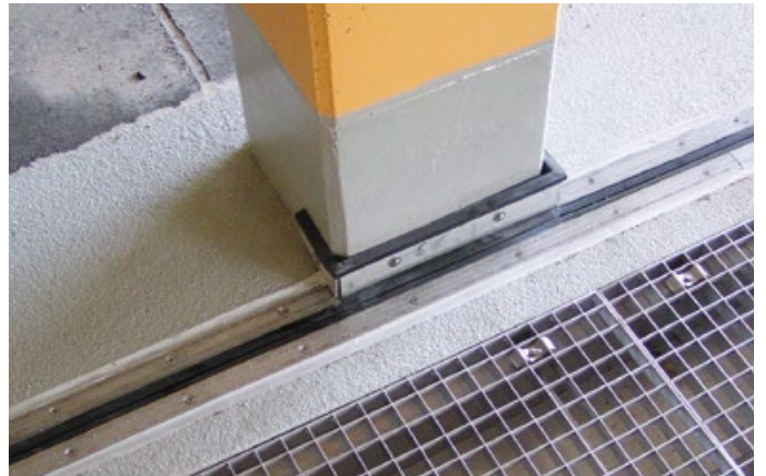
Parking garage Annaberg, Germany – FP 90
