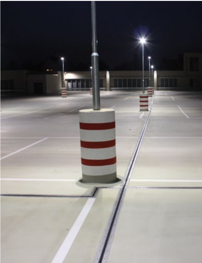
Parking deck shopping mall Dresden, Germany
